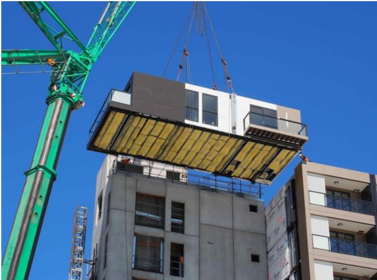
Figure 1: A building constructed using pre-fabricated units<sup>2</sup>.
